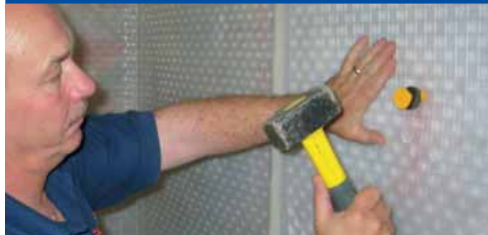
Or the Oldroyd Xv System (applied using sealed fixing plugs)...
