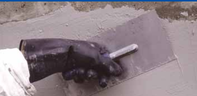
Either the Vandex System being applied by trowel...
